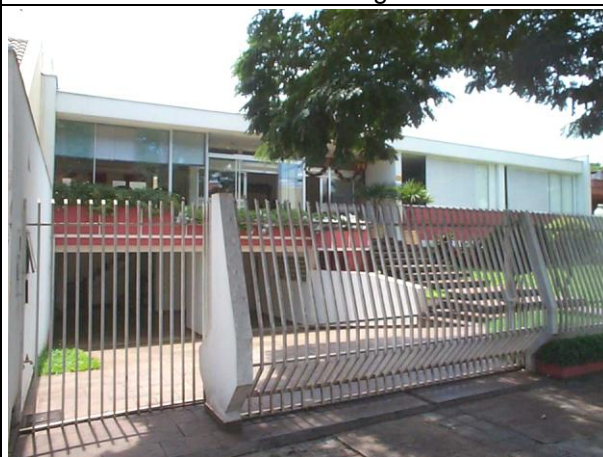
Rua Alfredo Pujol, 416
